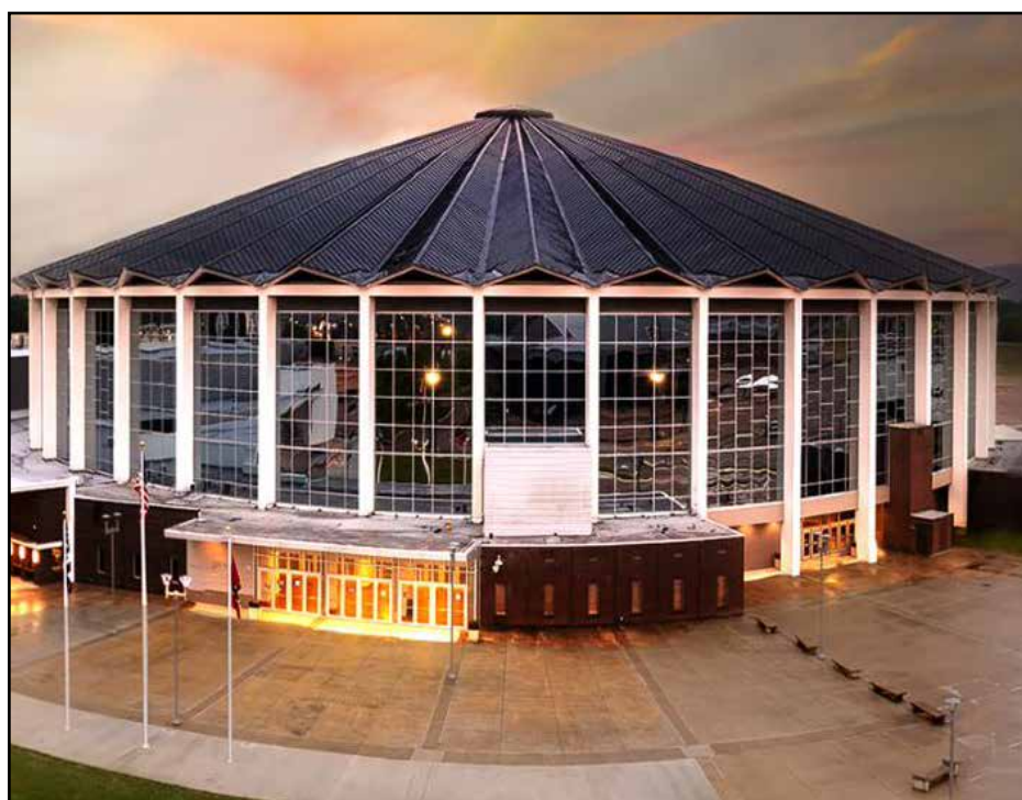
In January 1995, the old familiar yellow and red trim and white roof Mississippi Coliseum was renovated to a sleek black and copper structure. After numerous roof leaks, etc., an $18.5 million project changed the face of the coliseum. It included removing and replacing the roofing with a new, faceted copper cone roof and large mirror-like reflective panels. (Photo by the Mississippi Fair Commission)
